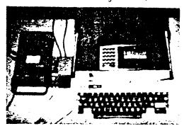
We have prototyped a "selectric" type keyboard to include all standard features plus custom engraved keys for the "command words" (i.e., GOTO, INPUT, etc.). This keyboard eliminates the need to press two keys to get one character.
